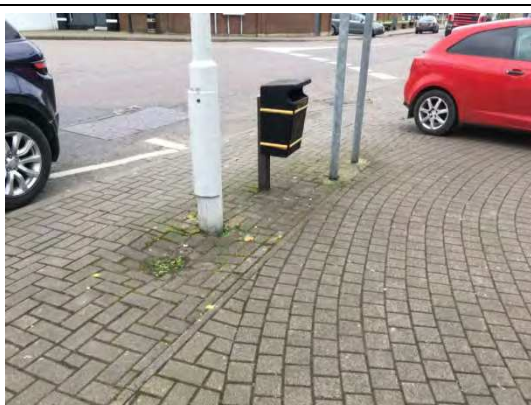
Dungannon Rd/The Square - highlights the present condition of the pavement including colour, vegetation group, and dips in the surface
