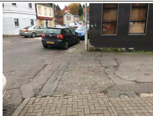
The Square - Section of footpath missing, asphalt surfacing is aesthetically poor with several areas of reinstatement visible.
