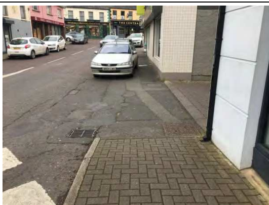
The Square towards Main St - There is currently no formal footpath provide in front of Donnelly McAleer Pharmacy. Asphalt surfacing is aesthetically poor with several areas of reinstatement visible.
