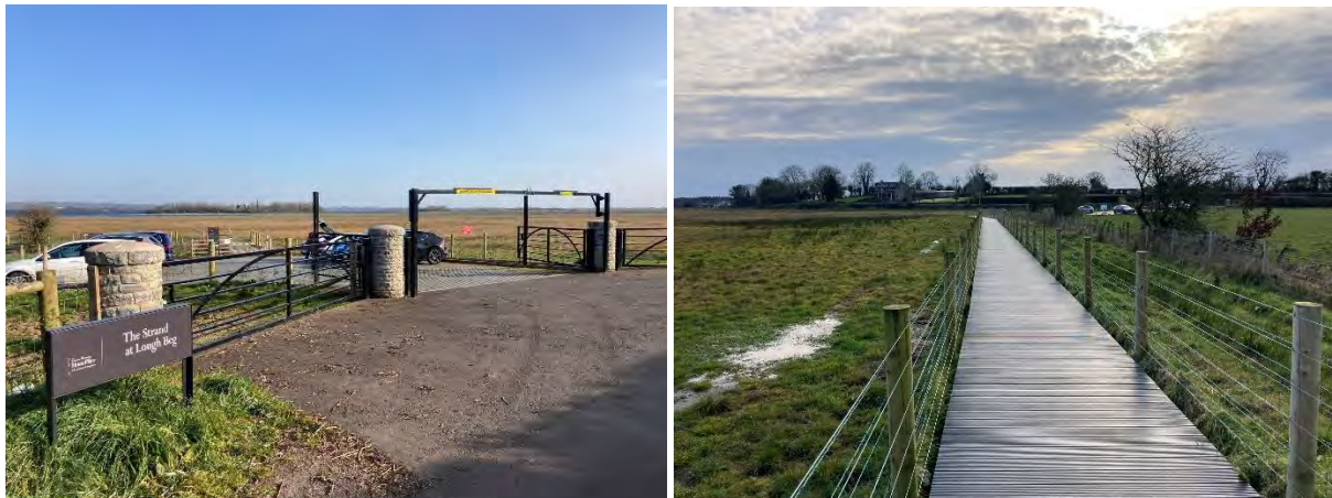
Figure 15 Boardwalk across wet grassland habitat at The Strand, Lough Beg
