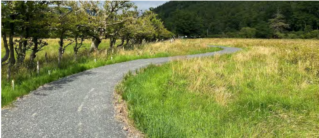
Figure 17 Raised causeway path construction and example
