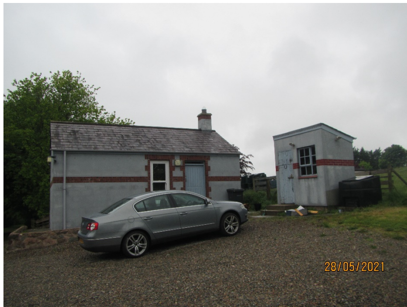
Figure 3 – snapshot of the building at the site
