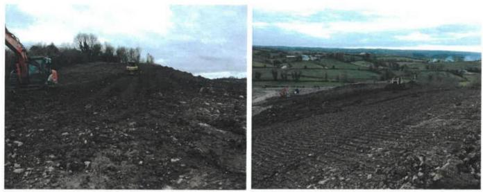
Pictures showing the Southern section of the site during grading of the soil stockpile area prior to covering with soil and tree planting.
