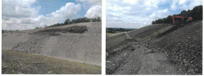
Pictures showing the final grading of the Cell 4 slopes which are now ready for either lining as a landfill cell or for landscaping. Slopes are to be seeded with wildflowers / grasses as an interim measure to reduce erosion.
