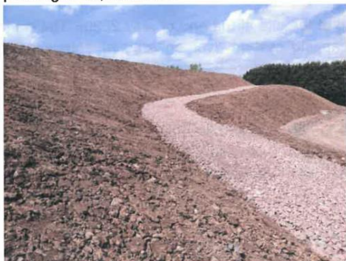
Pictures showing a before (left) and after (right) comparison of the finished cap following seeding with wild grasses on the Eastern flank of Cell 1 adjacent to the Site Office and Household Waste Recycling Centre.
