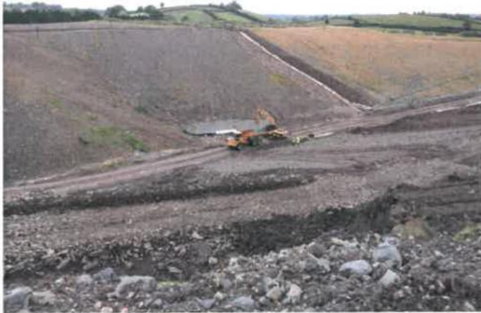
Pictures showing a before (left) and after (right) comparison of the Western Flank of Cell 4 following capping and seeding with wild grasses.
