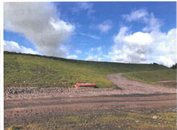
Pictures showing a before (left) and after (right) comparison of the finished cap following seeding with wild grasses on the Eastern flank of Cell 1 adjacent to the Site Office and Household Waste Recycling Centre.
