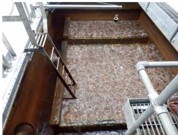
Figure 2.2: Backwashing a Filter
