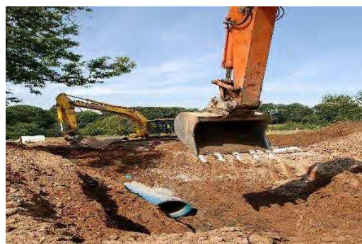
Figure 2.7: New mains installation
