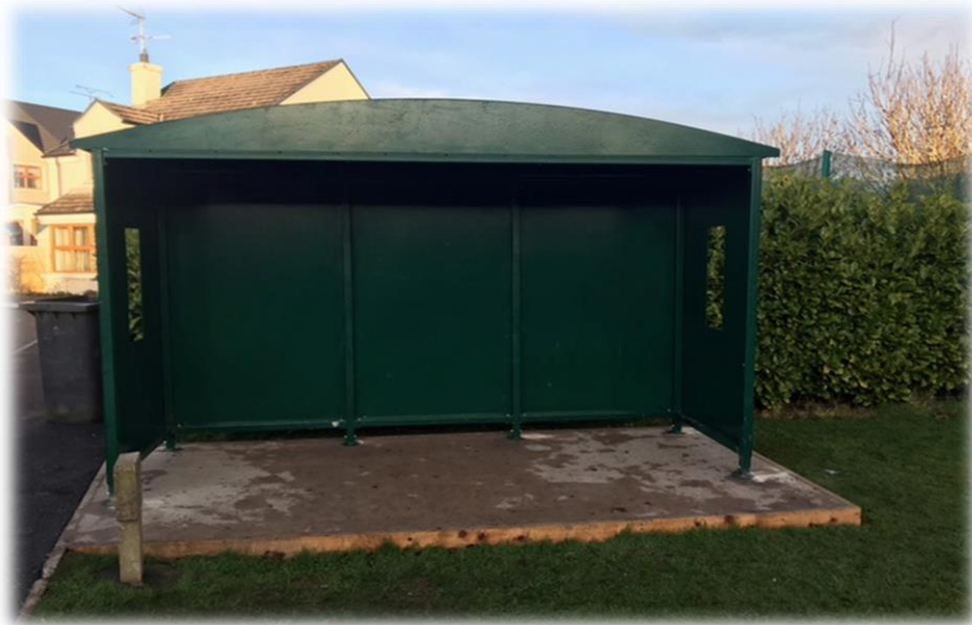
Newly installed shelter at Millview, Dunnamore
