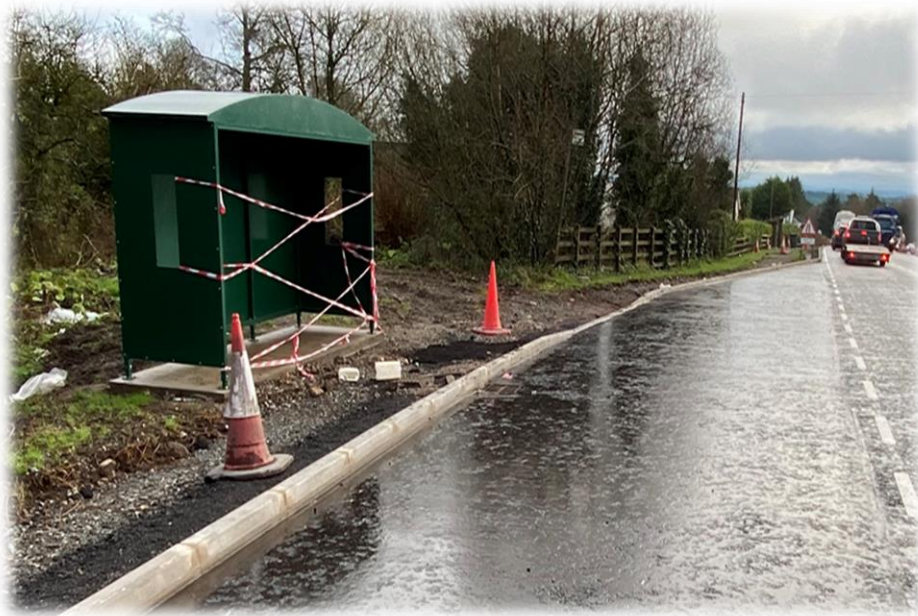
Newly installed Bus shelter at Omagh road, Ballygawley. DFI (Roads)
