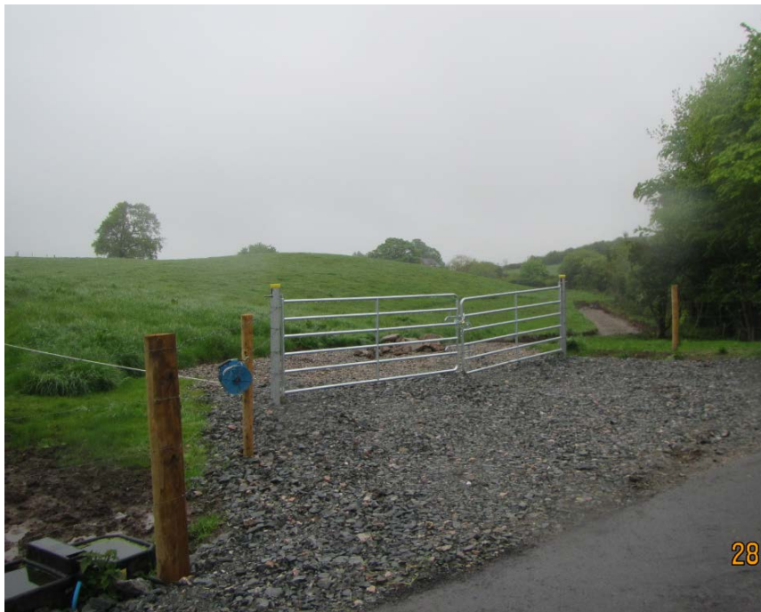
Figure 4 – Photograph of the access
