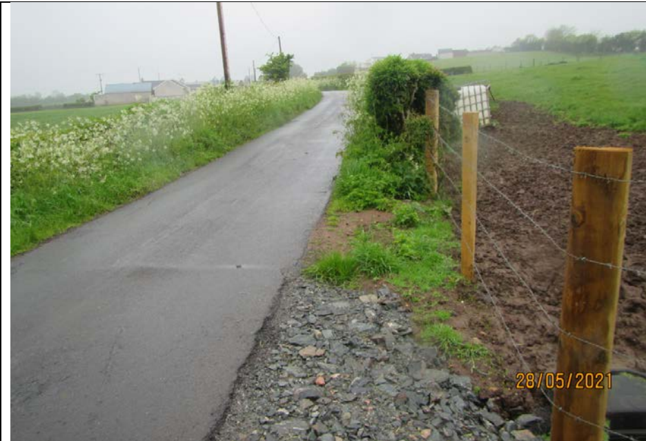
Figure 3 – Photograph to show the land cleared within the west splay
