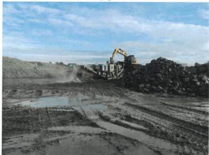
Pictures showing the rock crushing process carried out by Contract Ground Services (left) and the grading of the southern side of the site into an even slope ready for top-soiling and tree planting (right).
