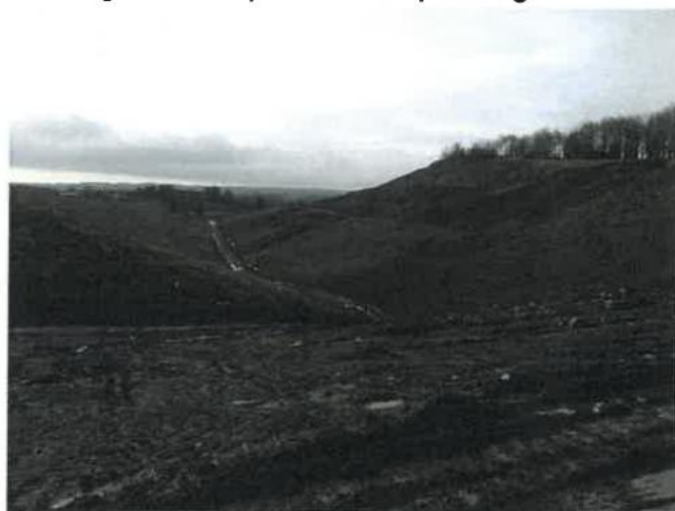
Pictures showing a before (left) and after (right) comparison of the western flank of Cell 4. The left picture was taken during the extraction of clay for capping Cell 1 with the right picture showing the bank being graded into shallower more stable slope.
