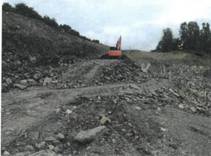
Pictures showing a before (left) and after (right) comparison of the Northern section of Cell 4 showing the grading of the steep rock faces and covering with soil prior to tree planting.
