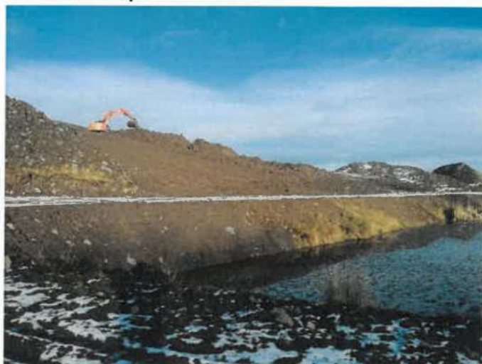
Pictures showing the rock crushing process carried out by Contract Ground Services (left) and the grading of the southern side of the site into an even slope ready for top-soiling and tree planting (right).
