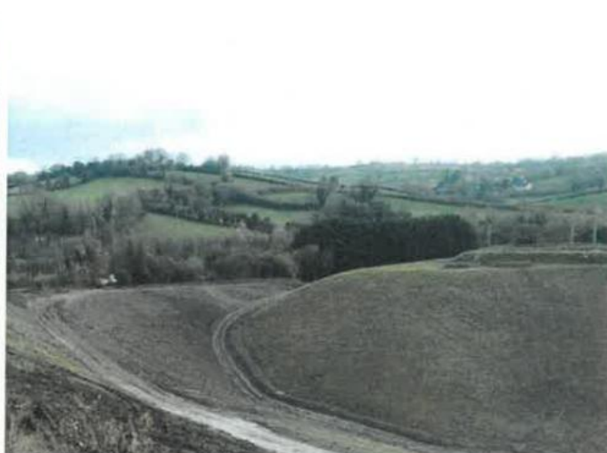
Pictures showing a before (left) and after (right) comparison of the Northern section of Cell 4 showing the grading of the steep rock faces and covering with soil prior to tree planting.
