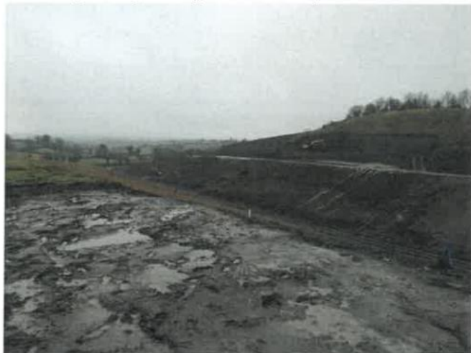
Pictures showing a before (left) and after (right) comparison of the western flank of Cell 4. The left picture was taken during the extraction of clay for capping Cell 1 with the right picture showing the bank being graded into shallower more stable slope.
