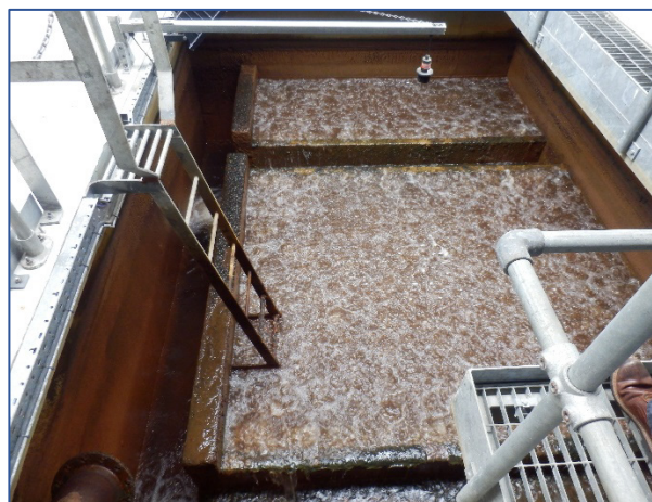
Figure 2.2: Backwashing a Filter
