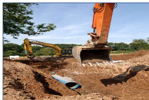
Figure 2.7: New mains installation
