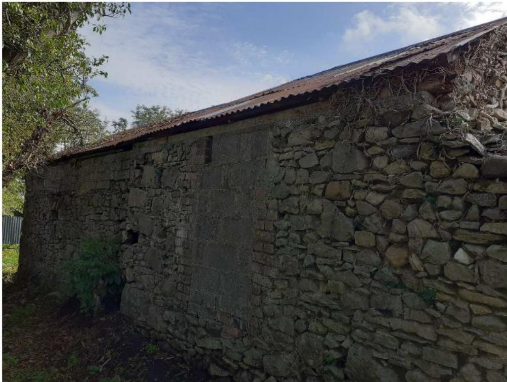
Figure 5 – Photograph of the rear of the attached building showing the windows built up
