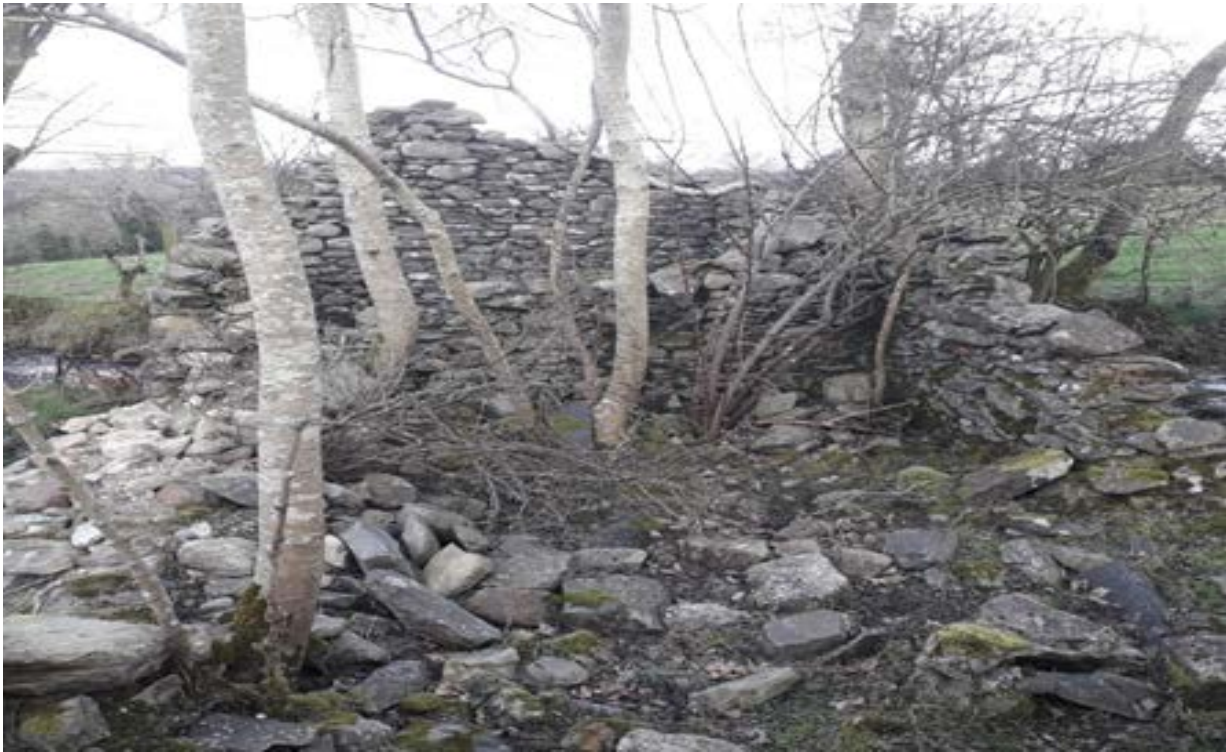
Figure 3. Clearly shows a significant part of the building having already collapsed with mature trees growing from within the building, which suggests this building has been abandoned for a very considerable period of time.
