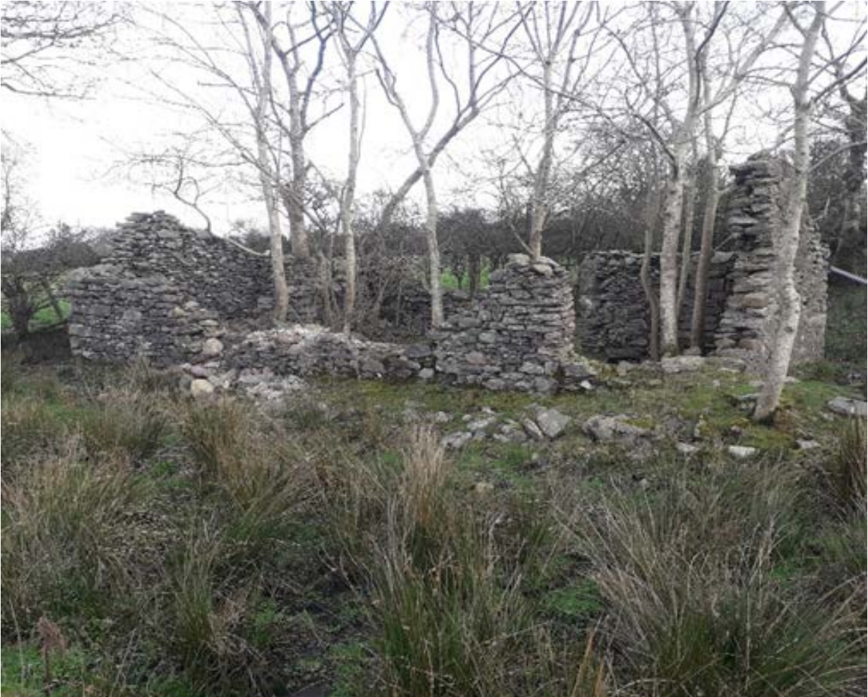
Figure 2. This photo shows the view from the front of building of one of the wallsteads. There is no evidence of any external window or door openings and the absence of roof. Observations made during the site inspection it was noted that there were no evidence of an internal fireplace, internal rooms and no evidence of any external chimney visible on the building.
