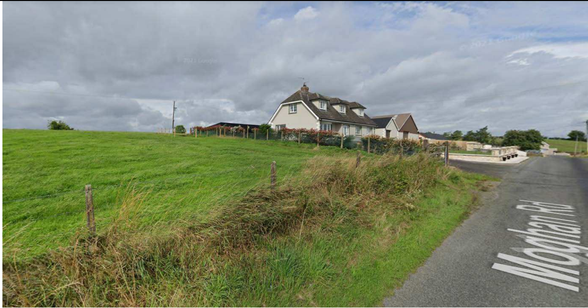
Fig 6 – dwelling and garage to side, viewed from south
