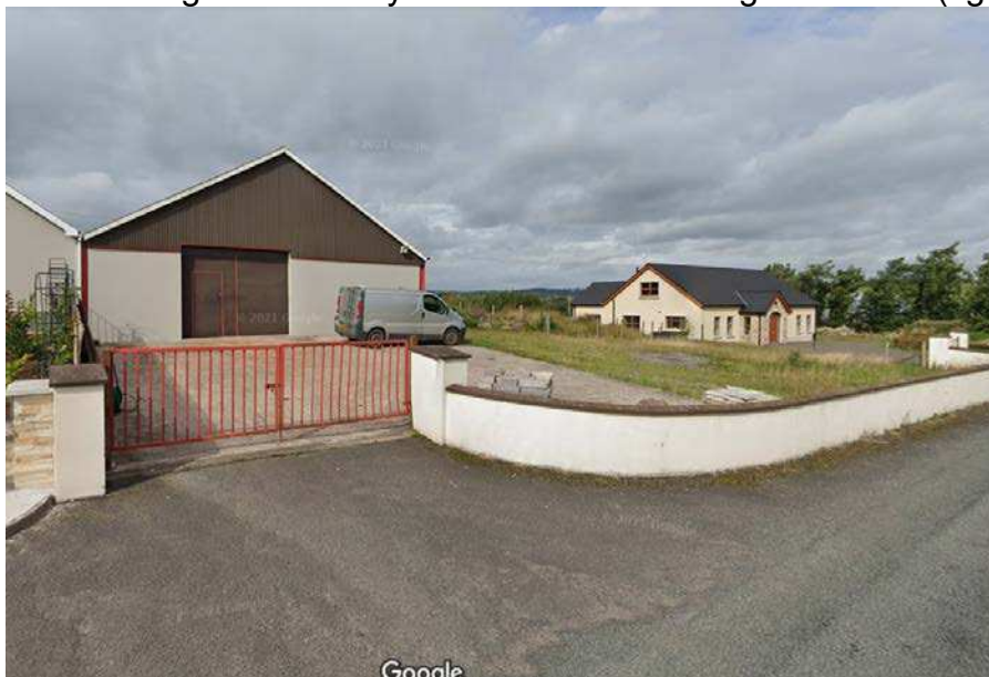
Fig 4 – shed and yard
