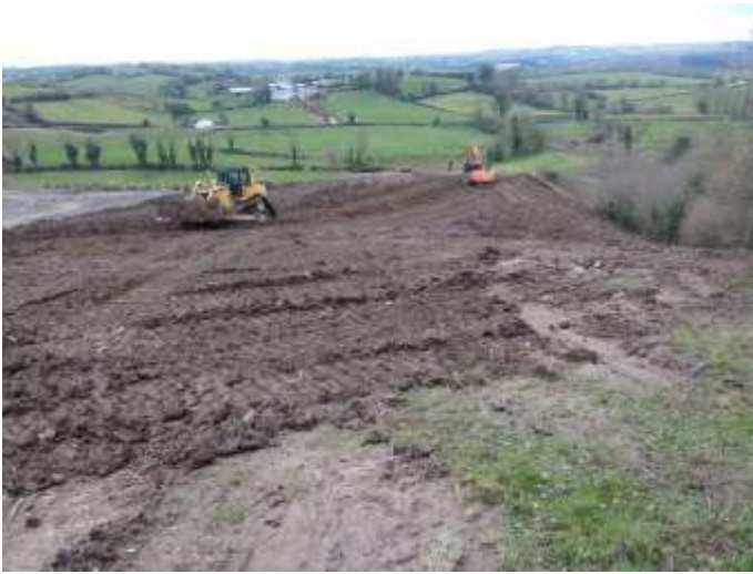
Picture showing the preparation of old clay borrow pit / stockpile areas with a bulldozer and tracked excavator (left). Picture showing the levelling of approx. 300mm of topsoil across the prepared slopes (right).
