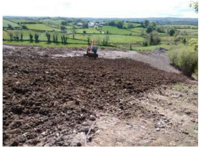
Picture showing the preparation of old clay borrow pit / stockpile areas with a bulldozer and tracked excavator (left). Picture showing the levelling of approx. 300mm of topsoil across the prepared slopes (right).
