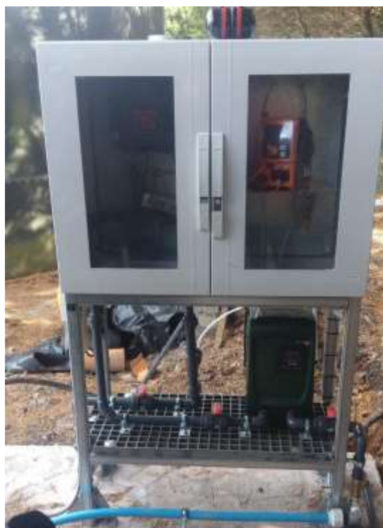
Picture 2: Continuous pH monitor and dosing pump.
