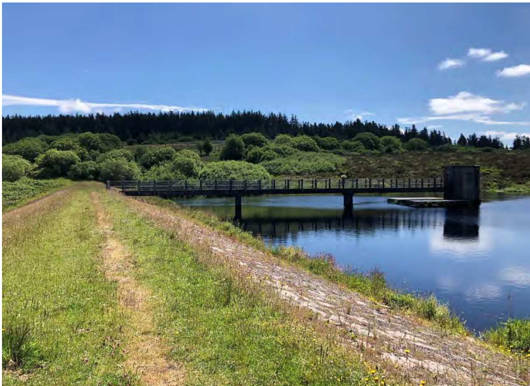
Figure 20 - Earth dam of the Upper Pond (Zone 2)
