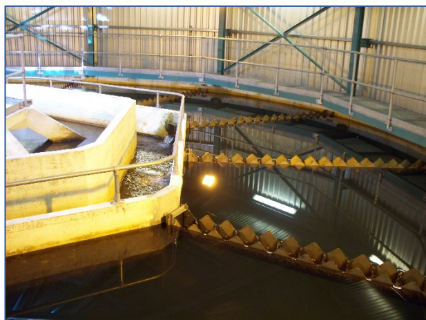
Figure 2.1: Clarification Stage
