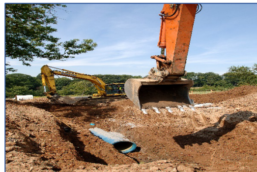
Figure 2.7: New mains installation
