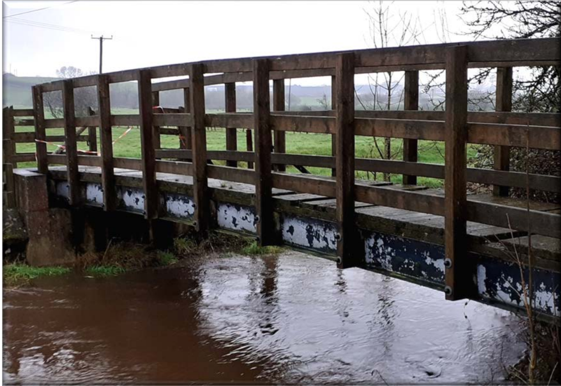
Fig 1 Side elevation of Bridge
