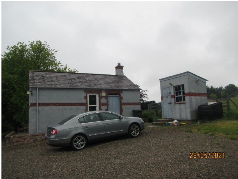
Figure 3 – snapshot of the building at the site
