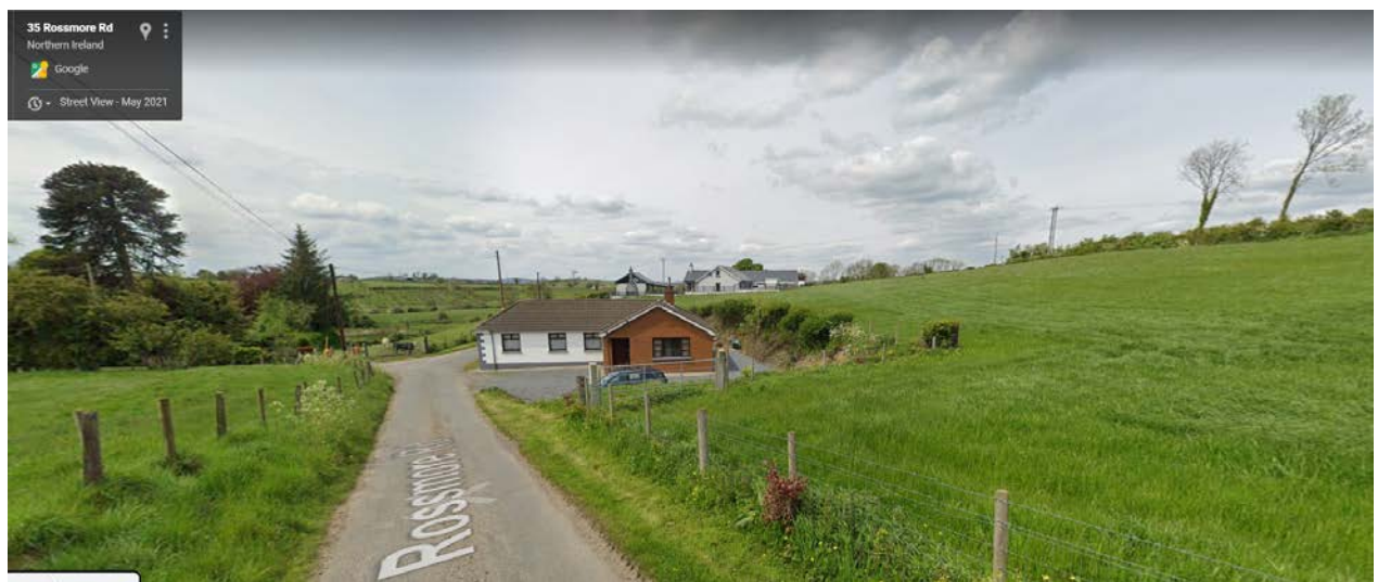
Fig 2 – No.24 is the dwelling with the red brick projection and the application site is land to the rear on higher ground.
