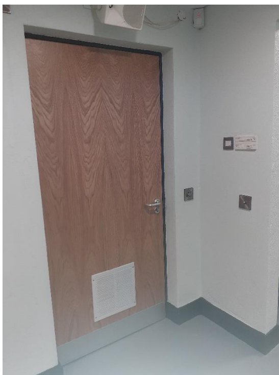
Widened door for wheelchair access and lowered light / control switches
