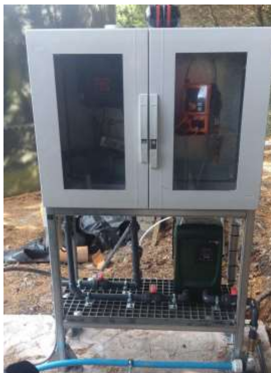
Picture 2: Continuous pH monitor and dosing pump.
