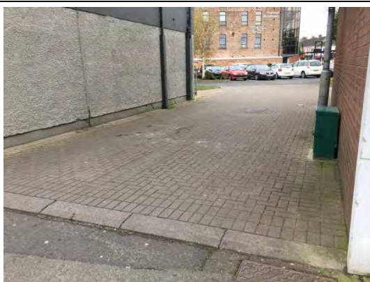
Access to Cornmill car park from The Square - No formal footpath provided to separate pedestrians from vehicular traffic
