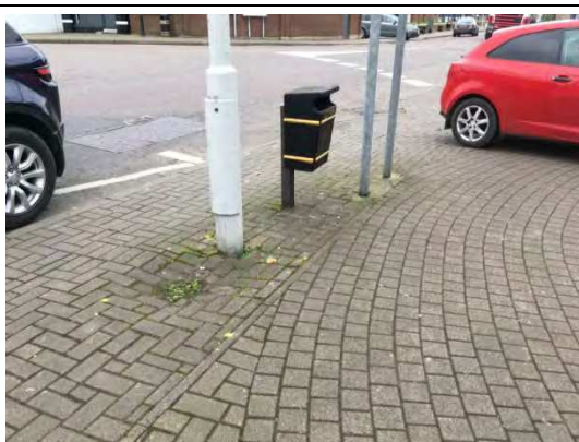
Dungannon Rd/The Square - highlights the present condition of the pavement including colour, vegetation growth, and dips in the surface
