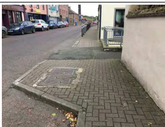
Main St - Section of footpath missing, kerb lines to not line up, causing ambiguity between carriageway and footpath
