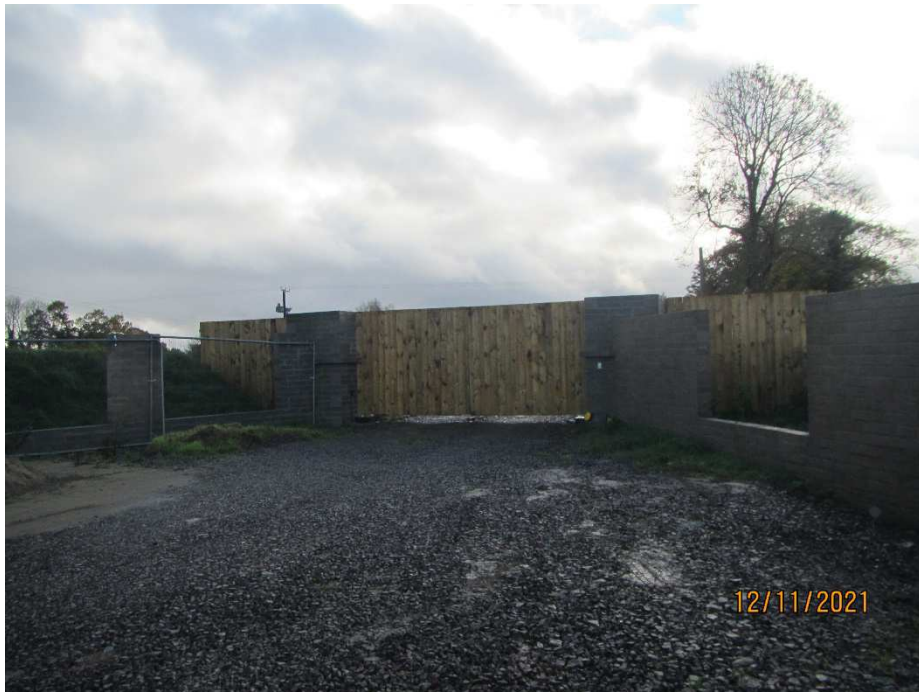
Figure 4 – Image from the site visit of wooden gates and pillars
