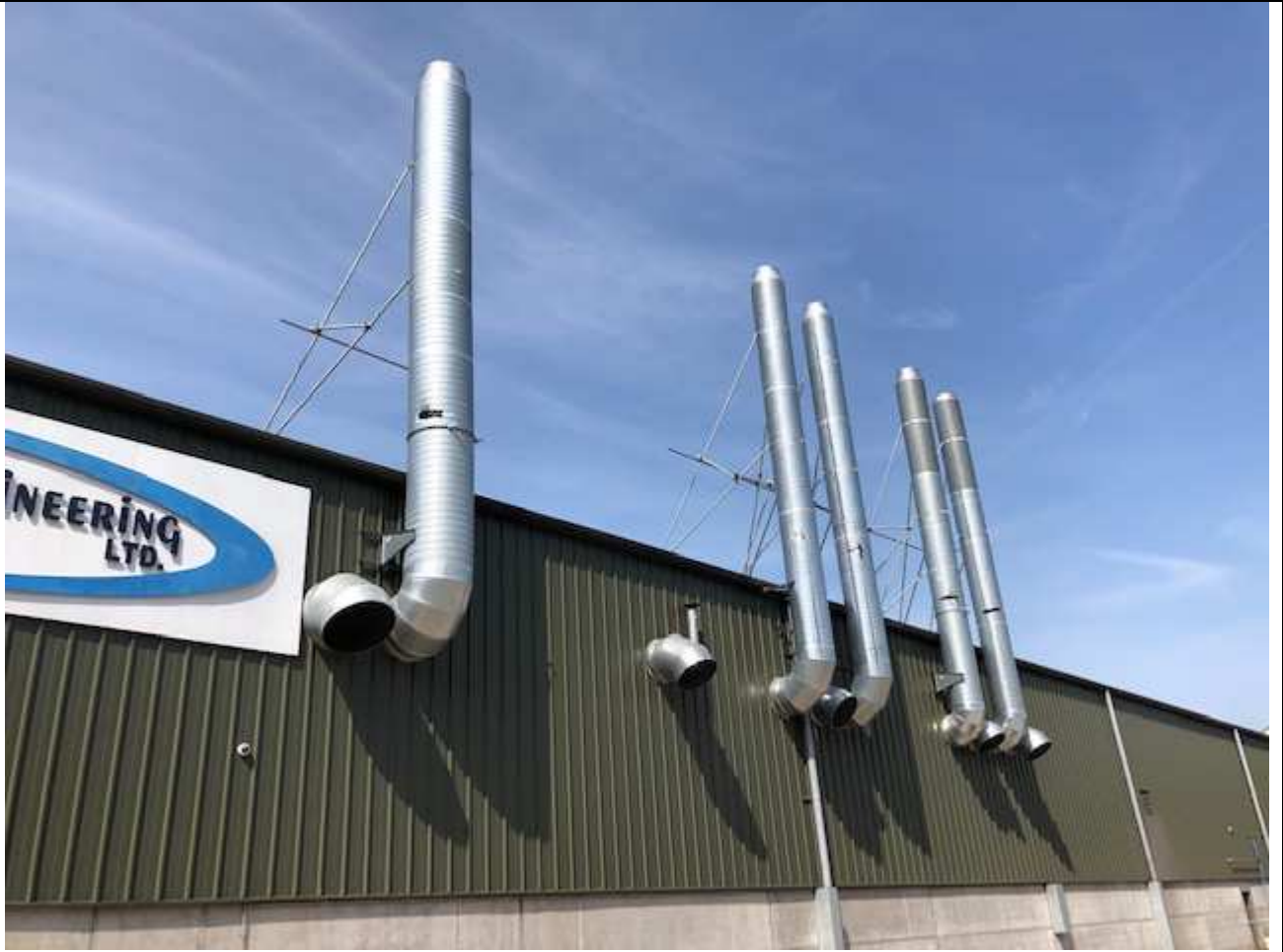
(stacks with support braces on side elevation)
