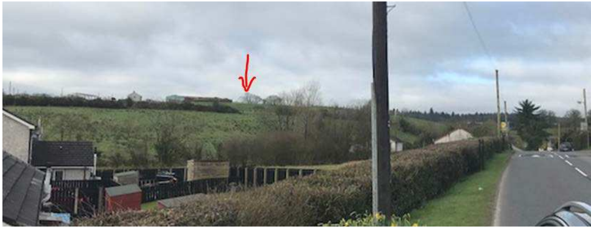
Photo B – View from Castlecaulfield - site identified in red in front of the trees, existing dwelling to left hand side with new pig shed under construction.
