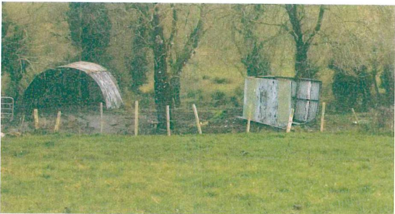
Fig.1 temporary structures constructed of timber and corrugated sheeting
