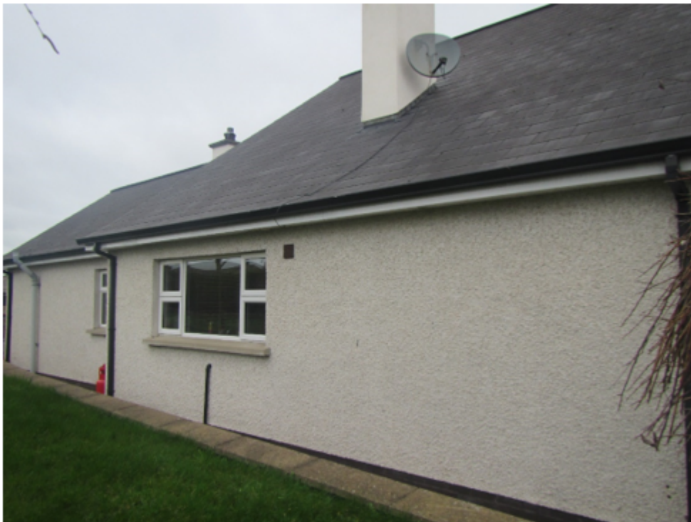
Figure 2 – View of No. 50 and the boundary of the site
