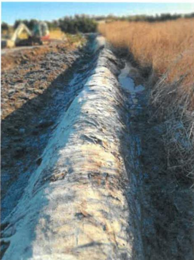
Picture 1 – Uncovering of existing bund geotextiles.
