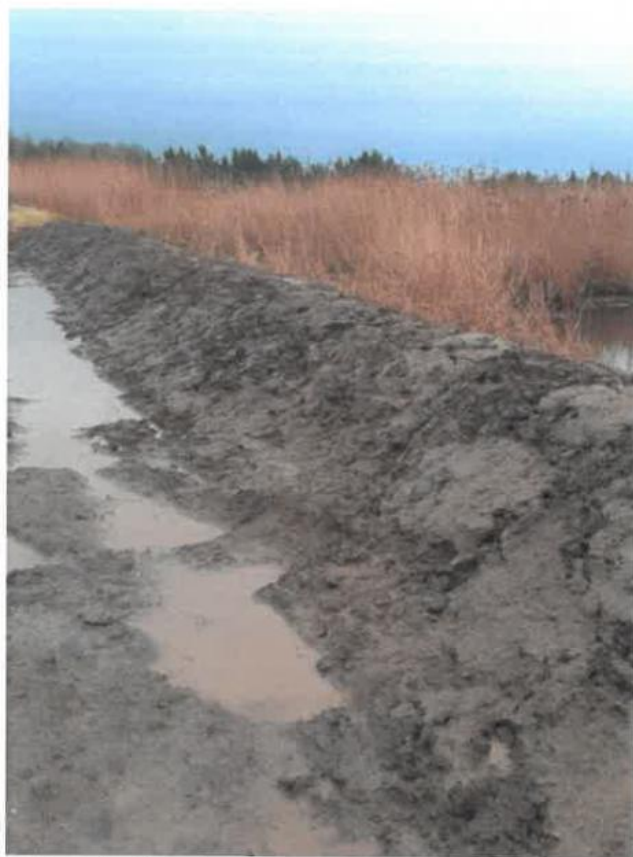
Picture 4 – Completed bund with soil applied.
