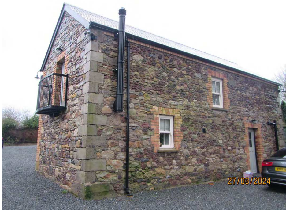
Image 2 - rear elevation, photo from further site visit dated 27/03/2024
