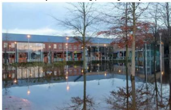
Flooding at the Linen Green in Moygashel in 2015
