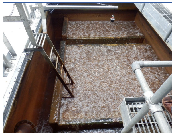
Figure 2.2: Backwashing a Filter
