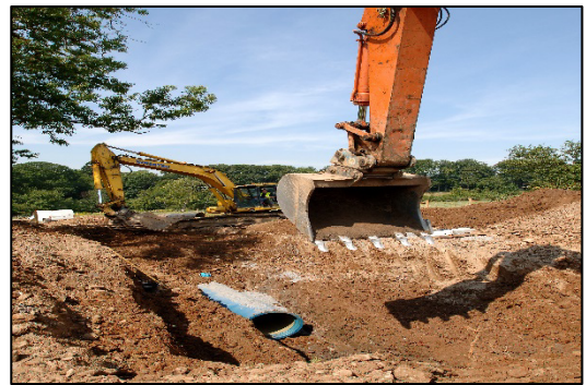
Figure 2.7: New mains installation
