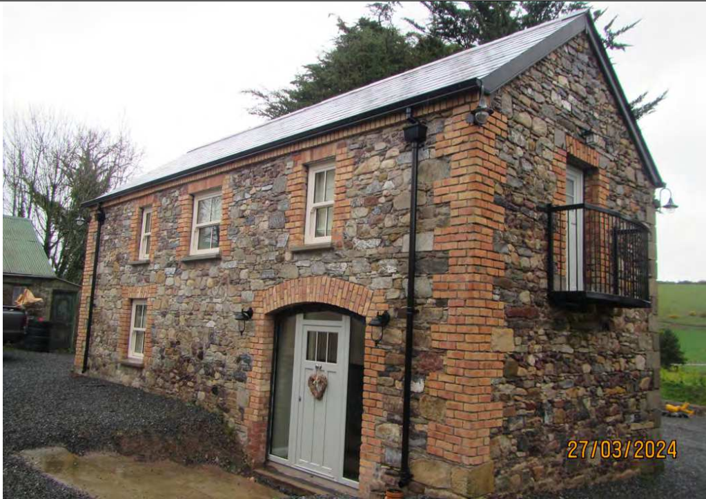
Image 1 – front elevation, photo from further site visit date 27/03/2024
