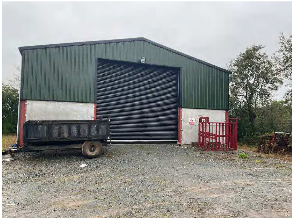
Figure 1 – Image from the site visit of the agricultural shed.
