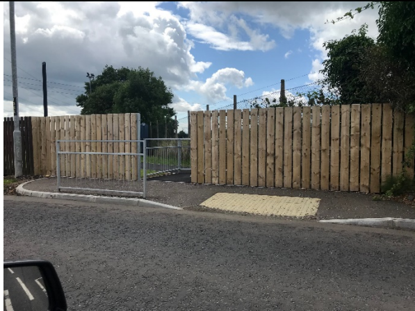
Fig 5 – pedestrian access as built to west (Coalisland side)
