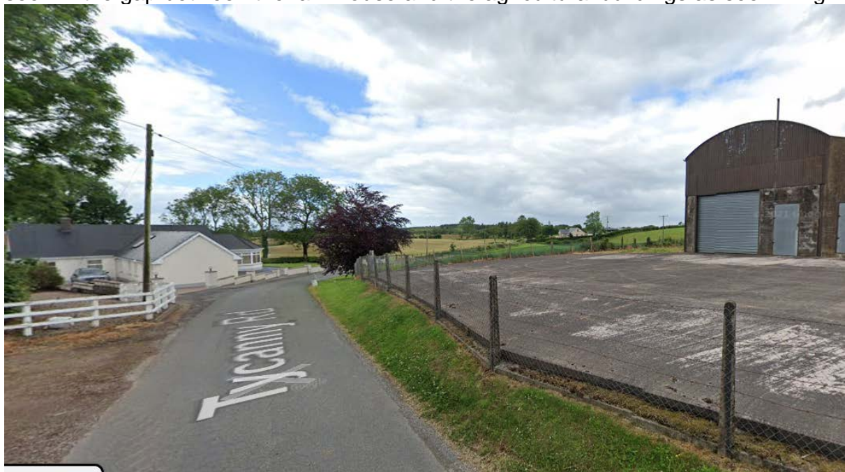
Fig 1 site from the north, dwelling located in area identified as red
