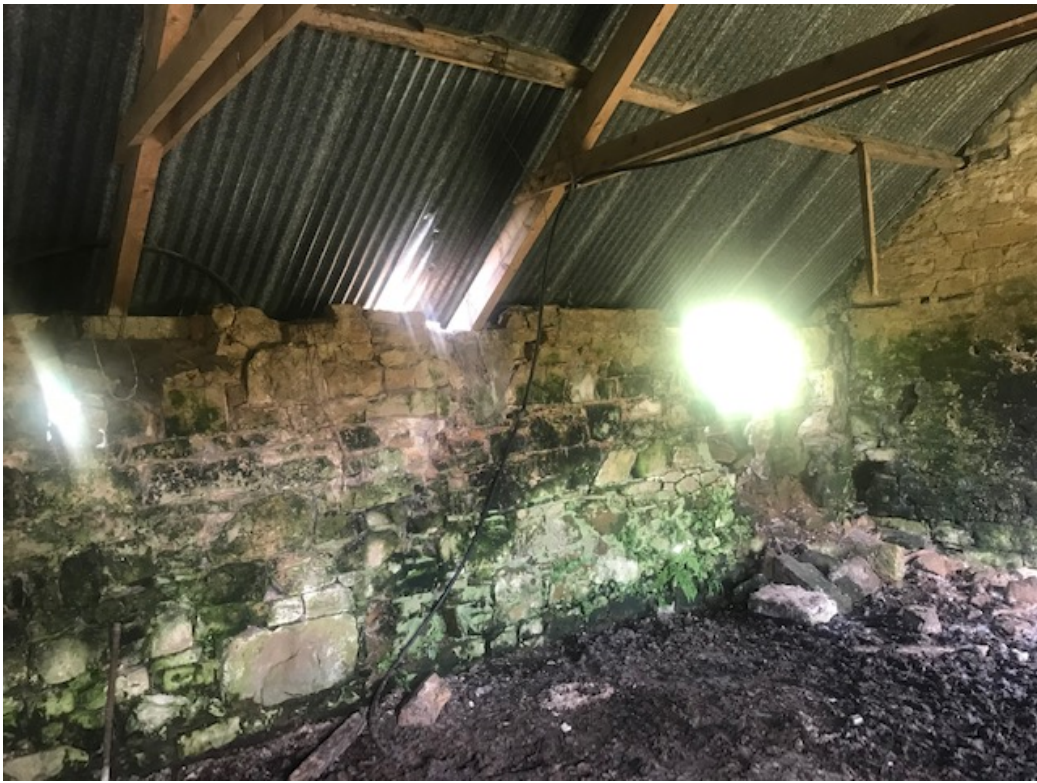
Photo 1 – internal picture from building
