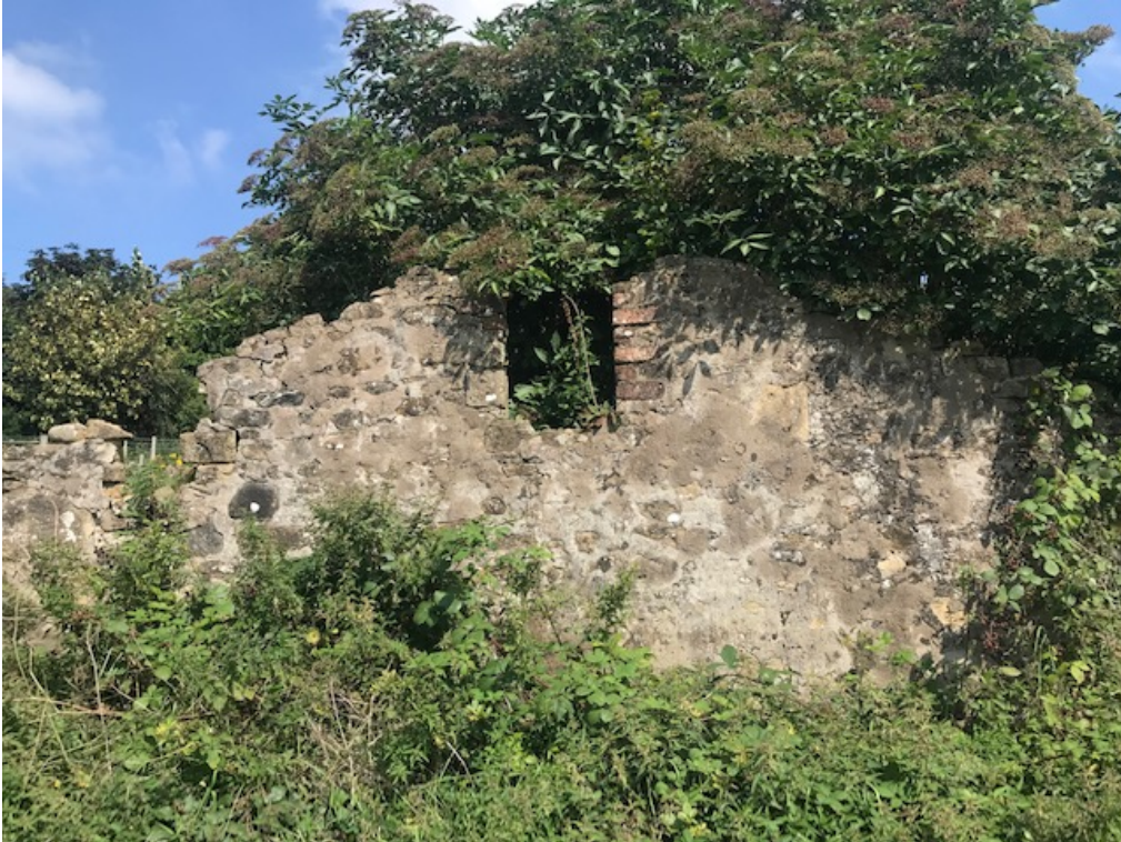
Photo 3 – External image of the building
