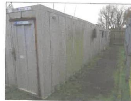
Existing Photos nts
