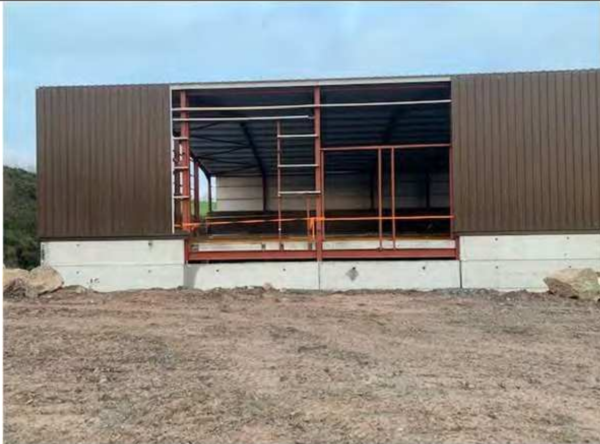
Level access into the first floor level
