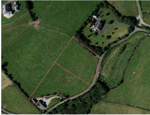
Figure 3 – Image of the site along the row
