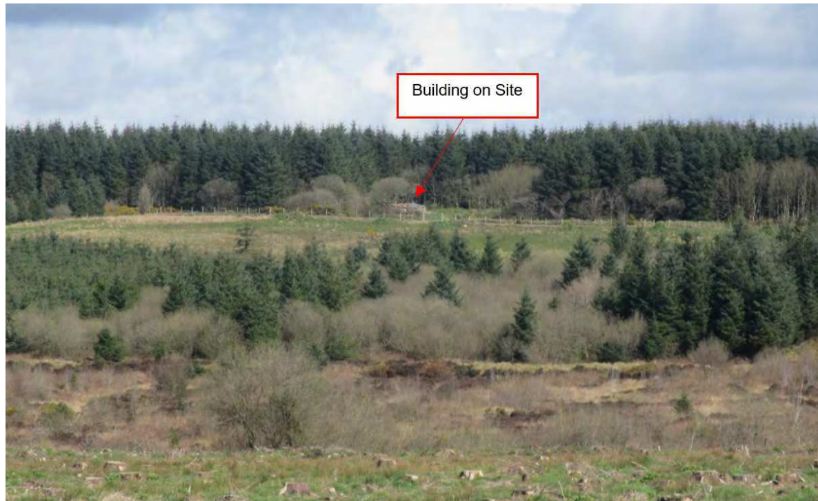
Fig 6: Photo of site from Barnagh's Road on the southwest approach to the site's access off Barnagh's Road
