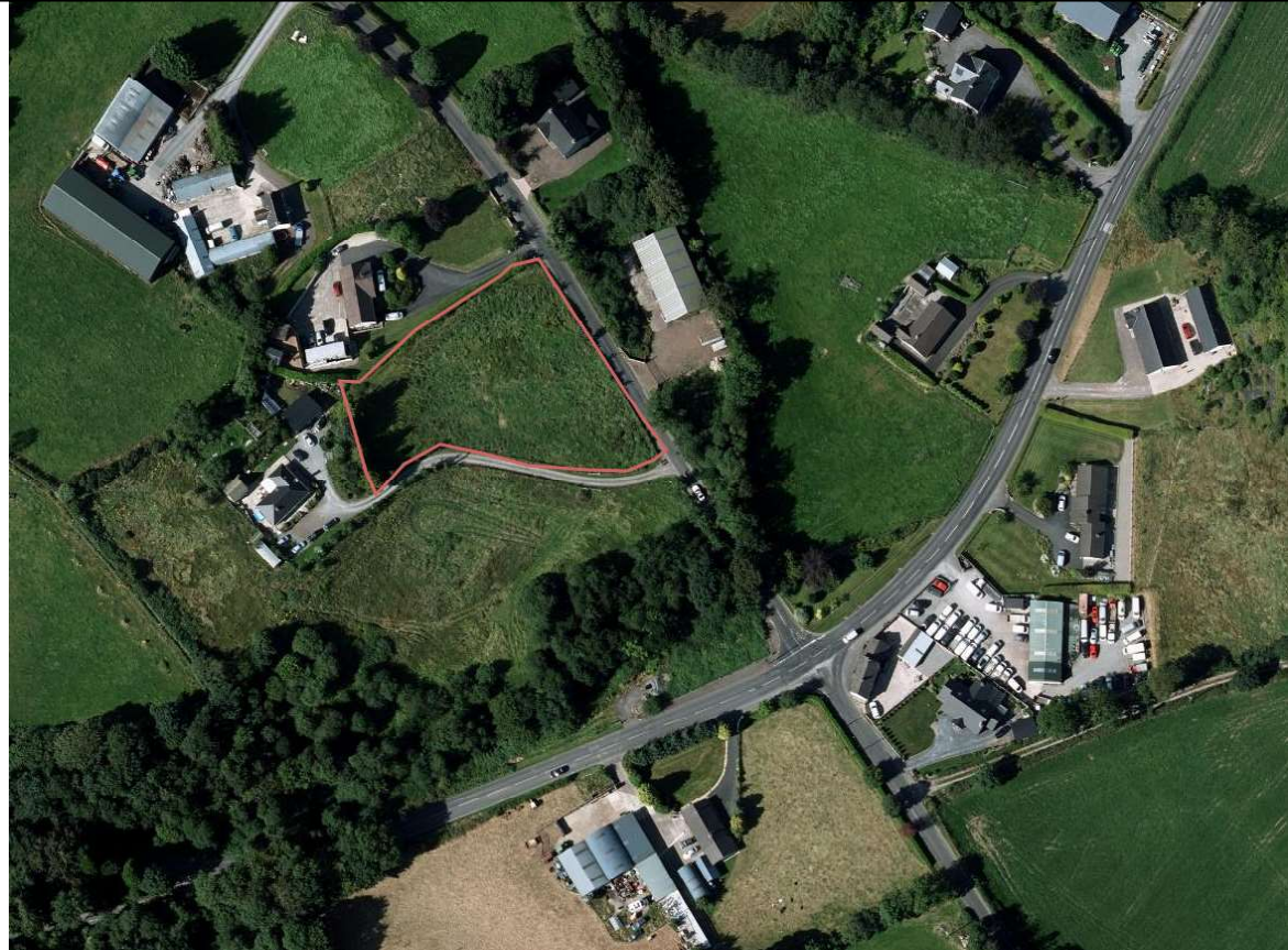
Figure 1 – Image of the site in the context of the surrounding area.
