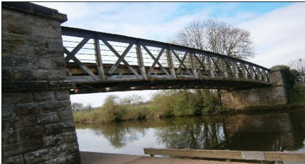
Verners Bridge, Dungannon
