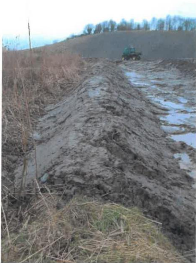
Picture 3 – Completed bund with soil applied.
