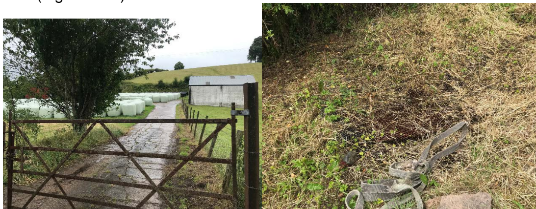
Fig 2 entrance to site with original building to right hand side, Fig 3 shows cover over septic tank both photographs taken 7 July 2023
