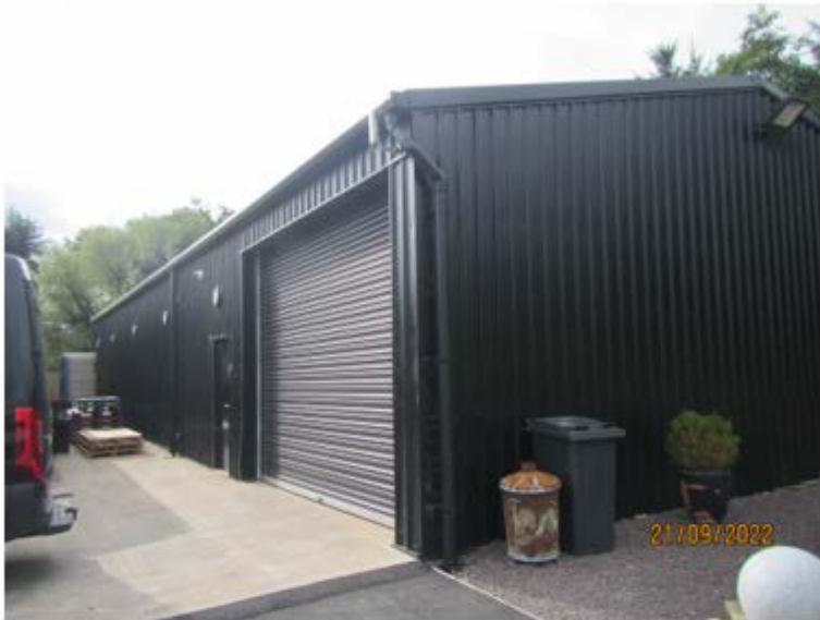
Figure 1 – Image of shed to be retained.
