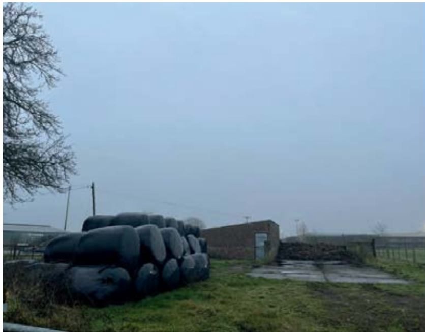
Existing building and silage clamp
