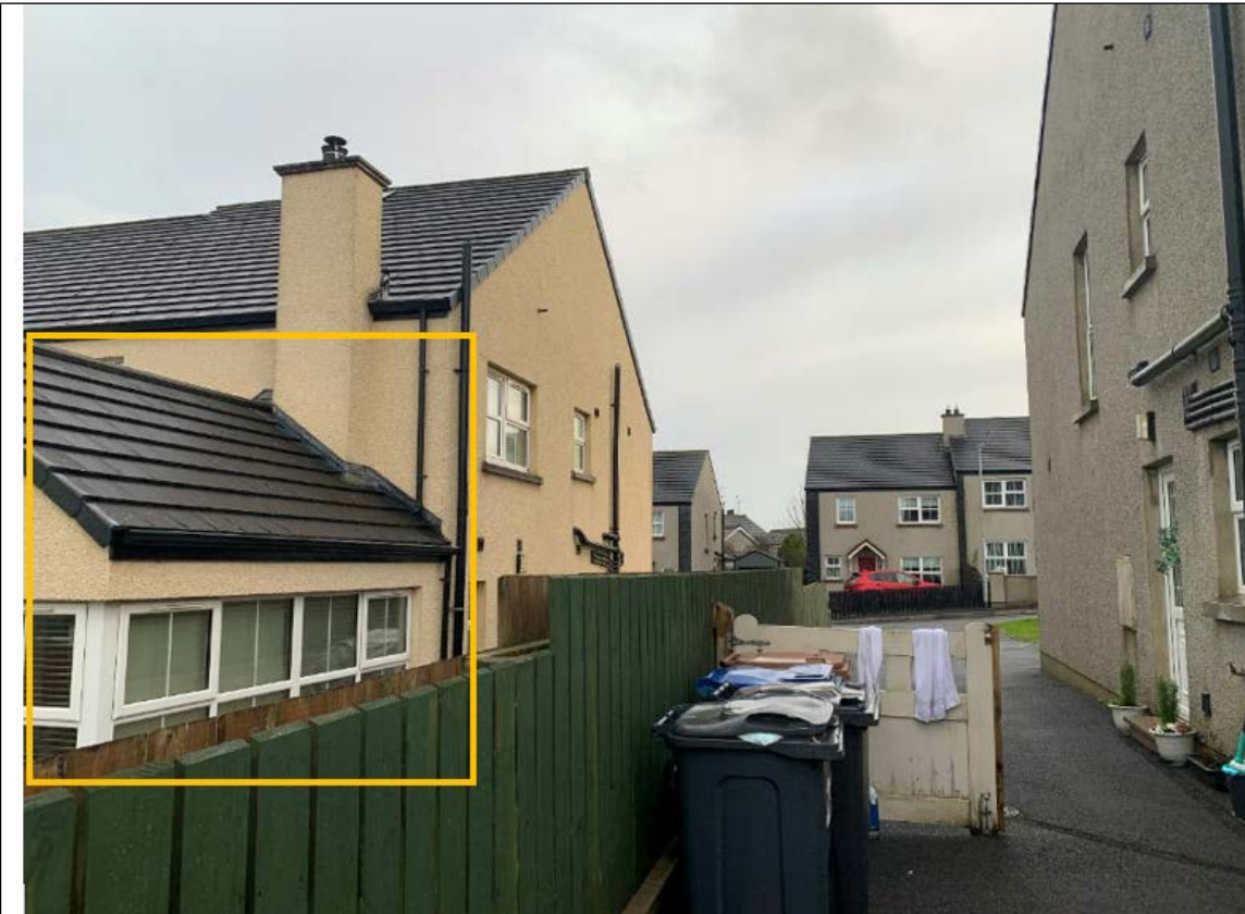
Fig 4: Photo showing the neighbouring property, no. 20 Ferny Ridge's sunroom.
