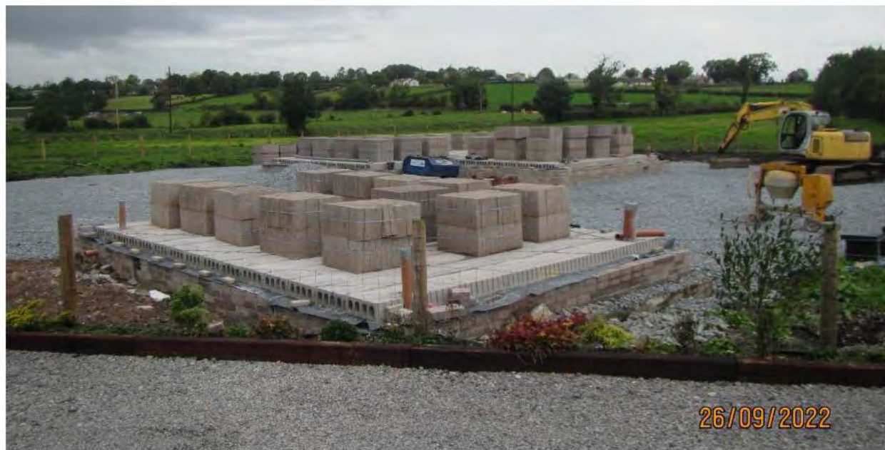
Fig 4: Photograph showing foundations of dwelling and garage on northern plot
