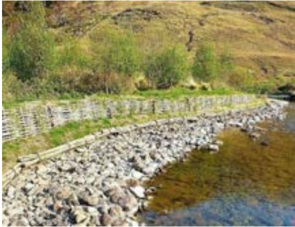
Figure 1: Bioengineering in Delphi to rehabilitate an eroding riverbank. (Rivus.ie).
