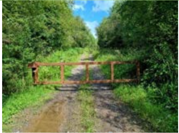
Figure 20: Section 3 existing FSNI gate
