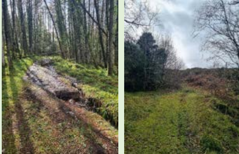
Figure 6: Upgrade surface of existing forest road and improve drainage
