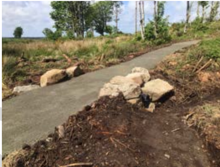
Stone headwall example side view
