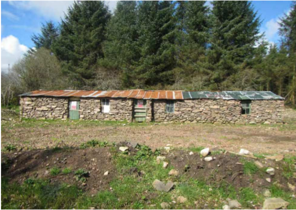
Fig 3: Photo of front (southeast facing) elevation of the building to be replaced
