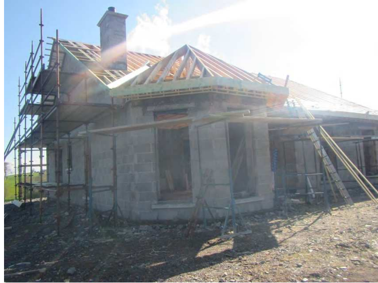
Figure 2 - Image of the front elevation of dwelling under construction.
