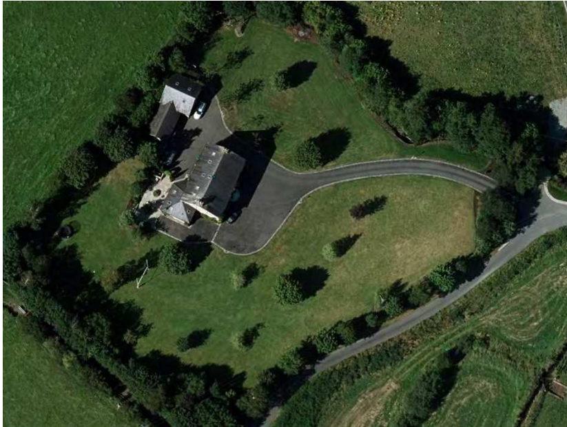
Figure 2 – Image of the dwelling at 65 Mullybrannon Road
