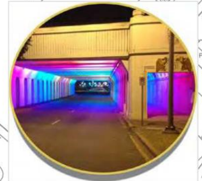
PEDESTRIAN UNDERPASS NEW LIGHTING BEECH VALLEY RD
