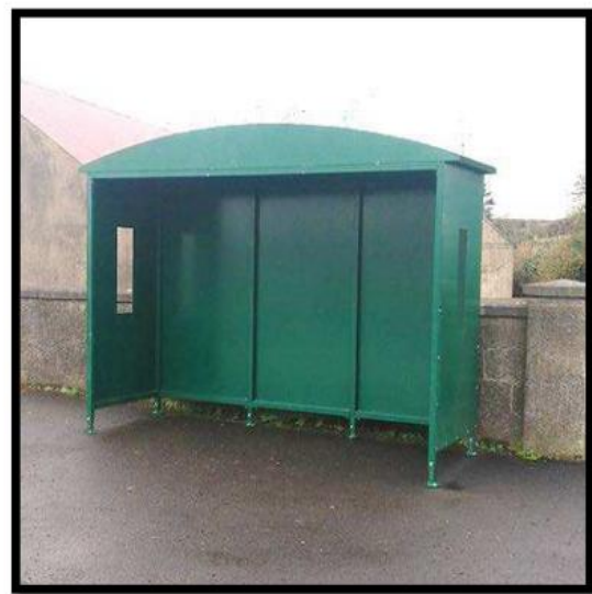
Example B , outside 30mph speed limits, painted metal shelter.
