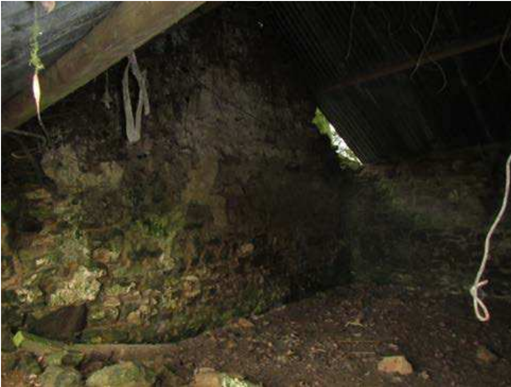
Rear wall with window opening blocked up
