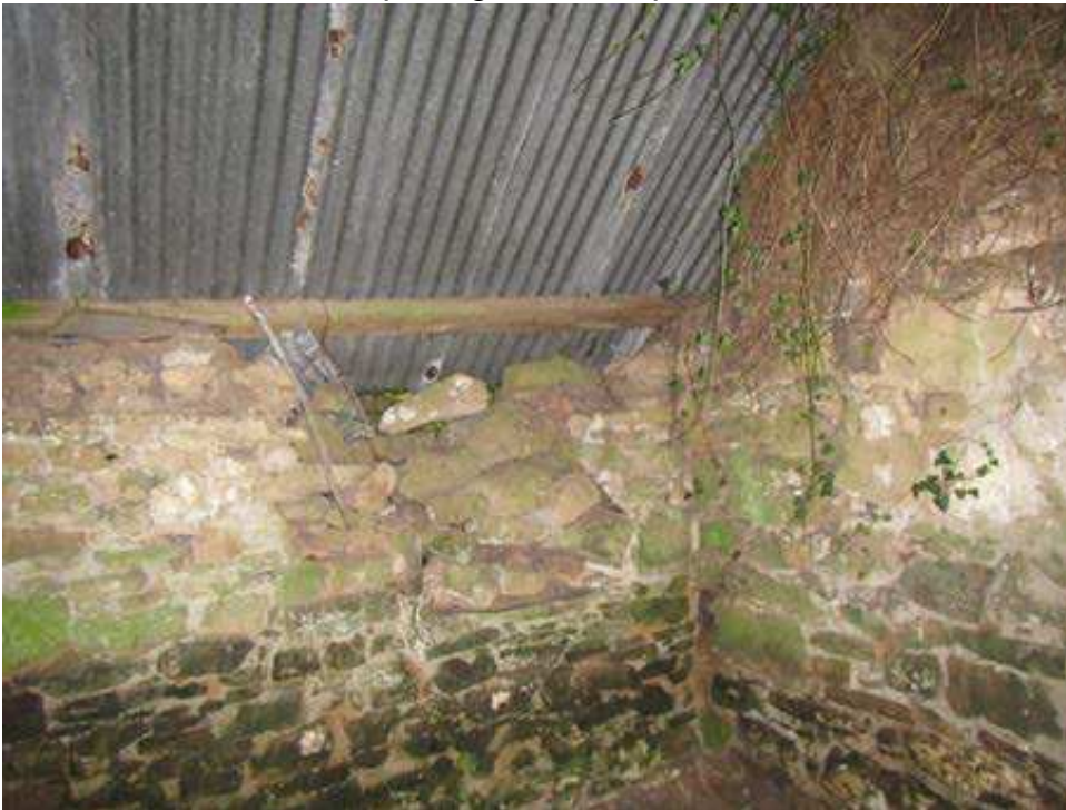
Rear wall with window opening blocked up
