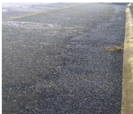
Carpark resurfacing and repairs
