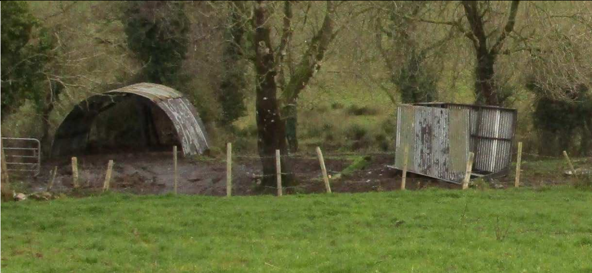
FIG. 1 Temporary structures constructed of timber and corrugated sheeting
