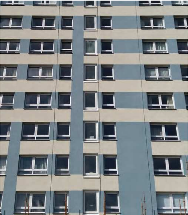
StoTherm Vario External Wall Insulation (EWI) at Carnet House
