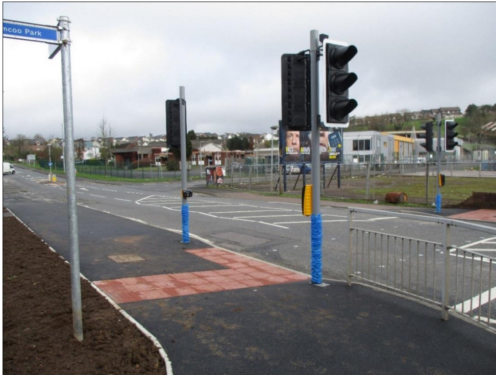
Toucan crossing and footway widening on A45 Oaks Road, Dungannon
