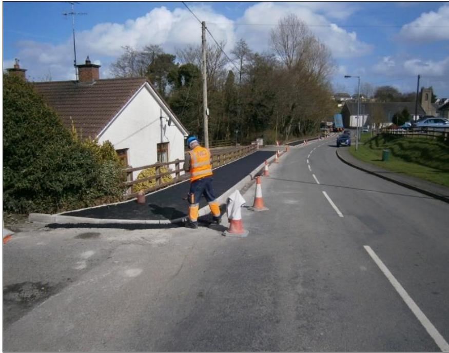
Footway extension with tactile crossing facility on Annaginny Road, Newmills
